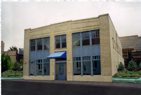
Paint and Awning Addition
