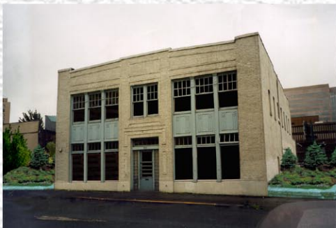
Stains on Brick Removed
