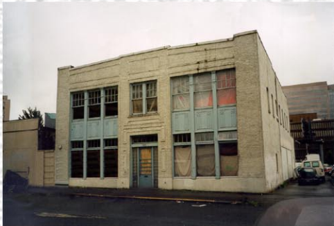
Telephone Pole Removed
