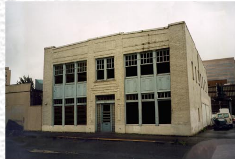
Windows and Curtains Removed
